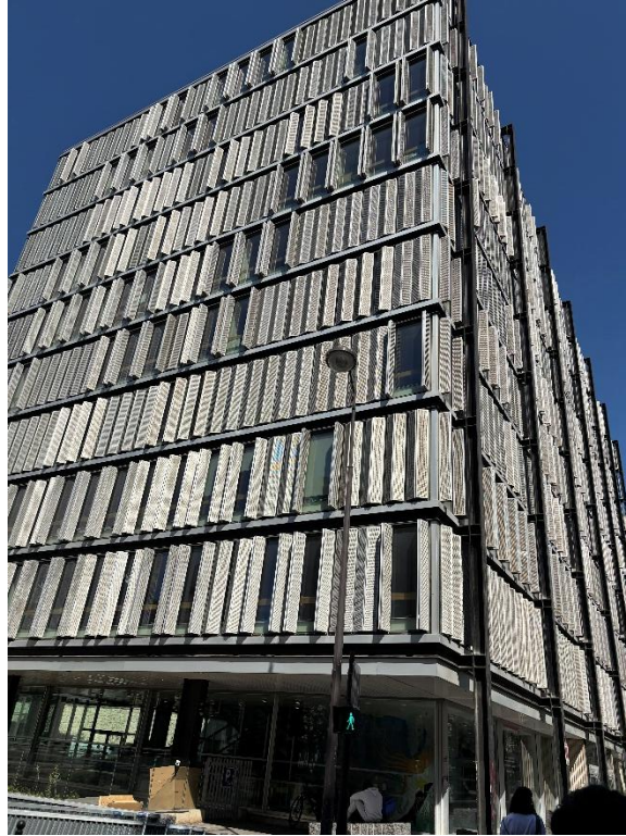
Figure 8 Modernist building with operable shutters. Photo courtesy of author.
