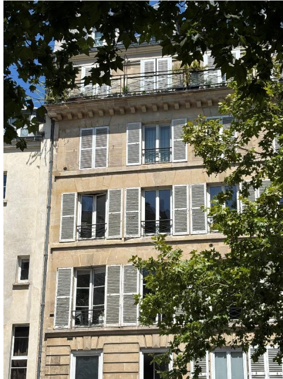
Figure 7 Building with operable shutters in the Latin Quarter. Photo courtesy of author.
