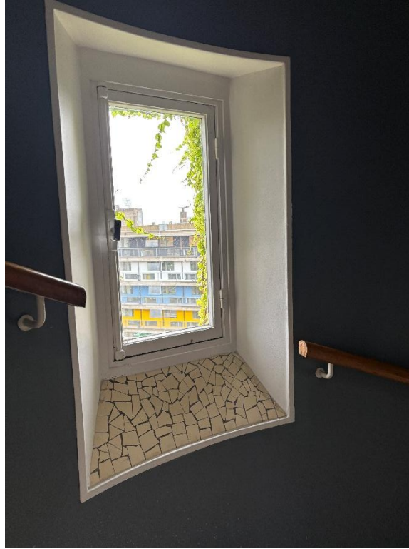
Figure 4 Splayed window in dorm stairwell. Photo courtesy of author.
